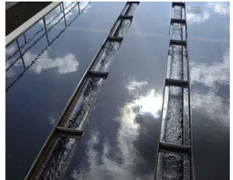
**Filtration** is the third stage of water treatment. The purpose of this stage is to remove the remaining suspended particles and dissolved constituents. This is accomplished by passing the water through a filter composed of different layers of sand, gravel and anthracite.
